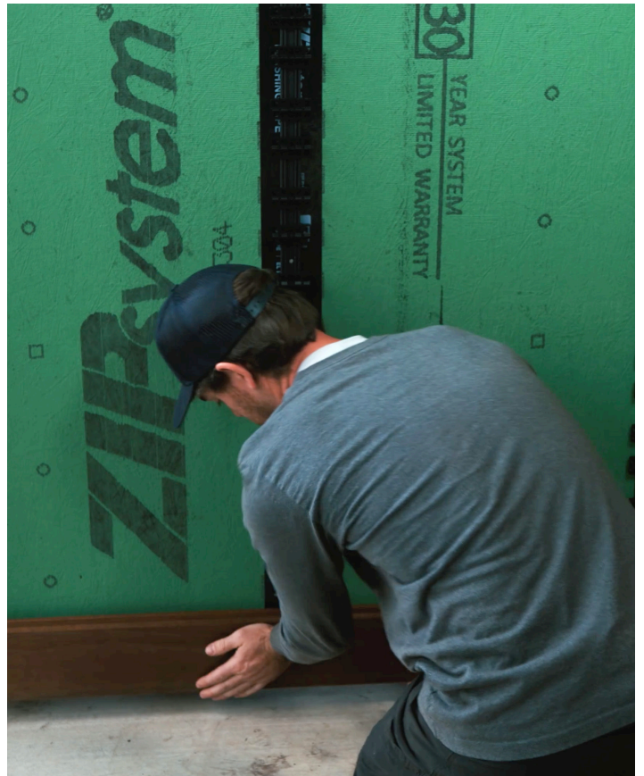
↑ Kebony® with Grad® Cladding installation
