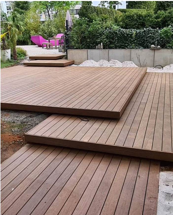
↑ Multi-level platform deck installation
